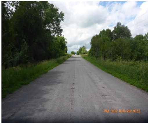
Figure 51 Images of Culvert No. C, Douro 9th Line
