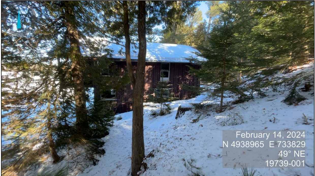
Photo 12 Slope face at western edge of boathouse.
