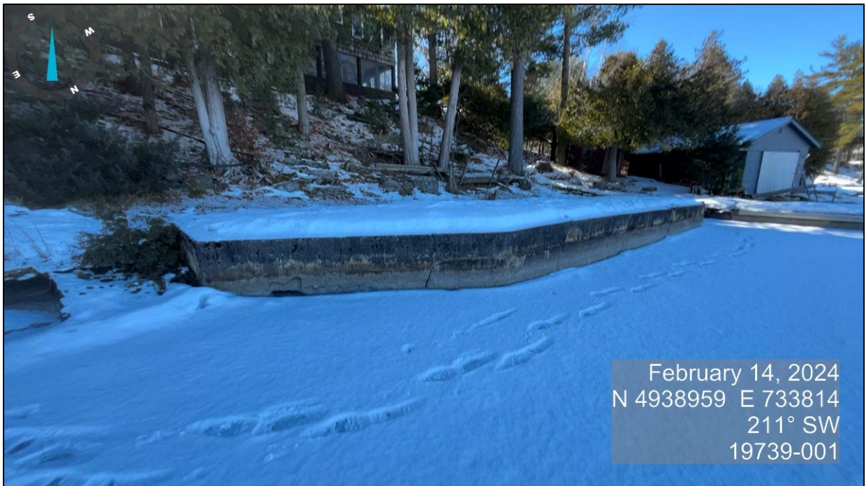
Photo 6 Concrete pier at the toe of the slope. Pier extends down to lake level.
