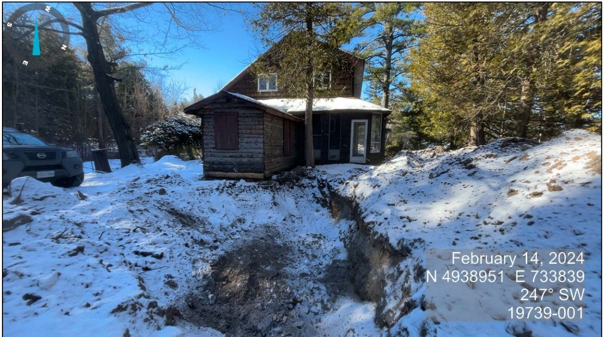
Photo 8 TP101-24. Table land above slope was excavated to expose bedrock for investigation.
